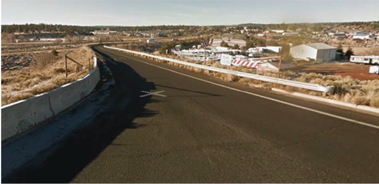
Figure 1-5: I-40 Westbound On-Ramp [1]
